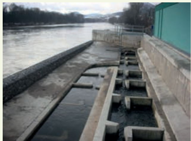
Picture 10 — Artificial fish crossing used mainly by faster fish species
