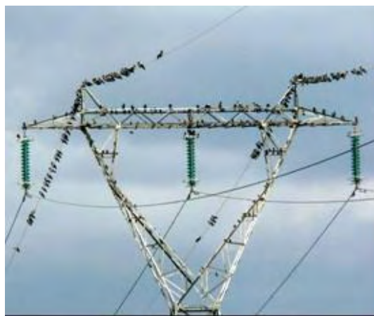
Fig. 7: Tralicci AT a Y.
