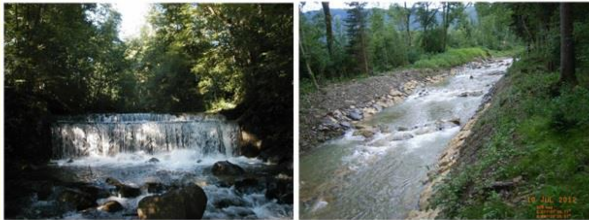
Illustration21 - Before and after; a 3m high check dam is replaced by a 120 m long ramp.
