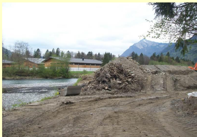
Illustration 25 -Example of works carried out on the oppositeriver bank to remobilize aggraded material.
