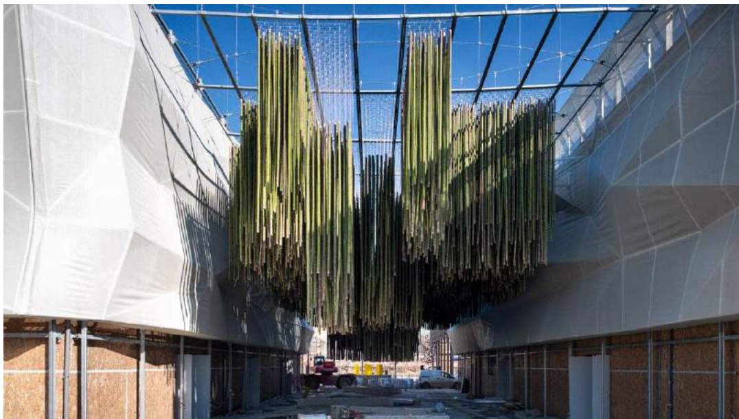
Figure 23. Building site of Islands Cluster: completion phases
