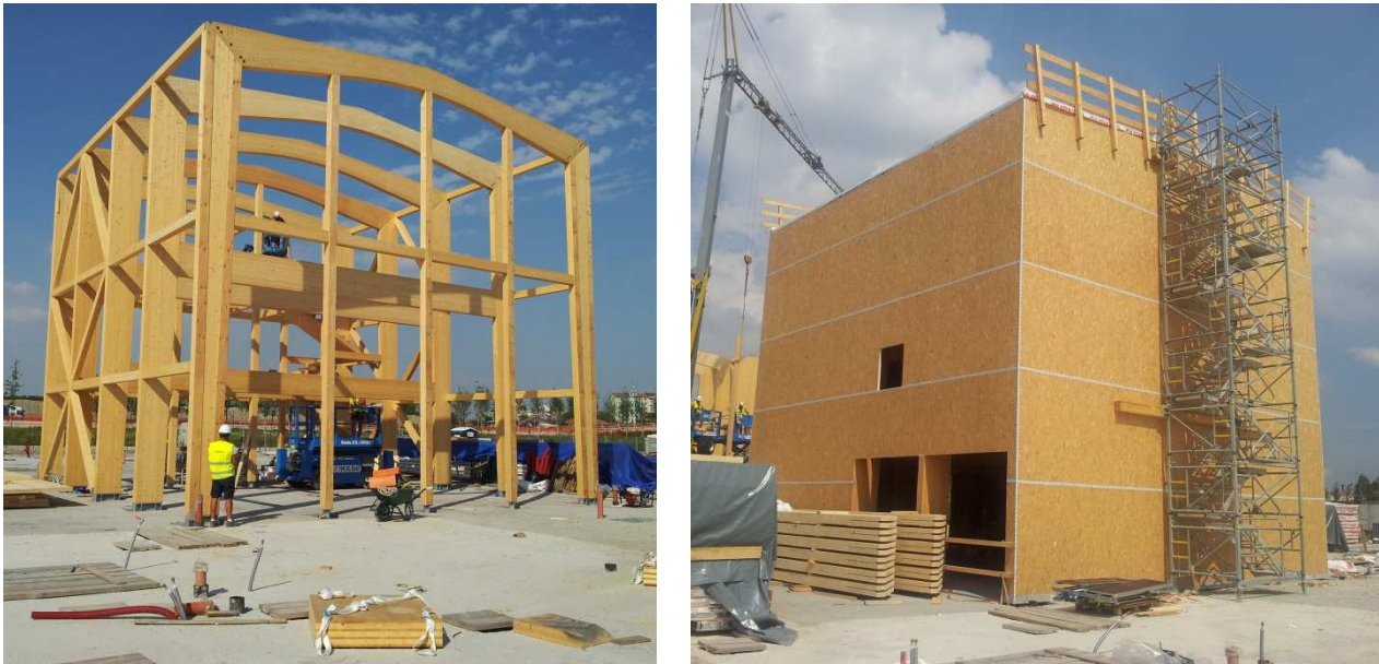
Figure 24. Cluster: laminated wood structure and standard modul
