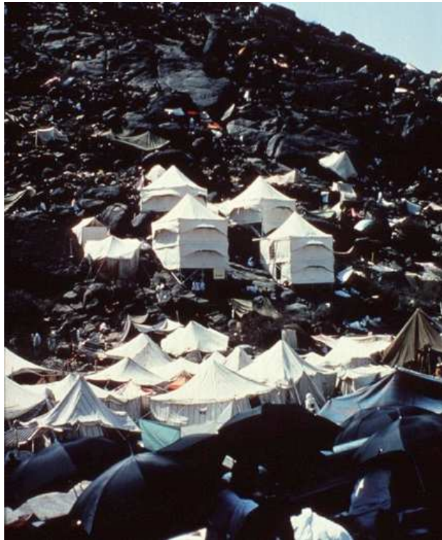
Figure 26. Frei Otto Design: two floors contemporary nomadic tent; aluminium structural frame and double layered transparent fabrics.
