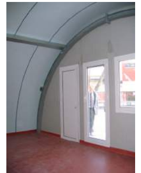
20. Inside plasterboard walls
