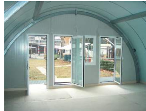
19. External wall in sandwich panels
