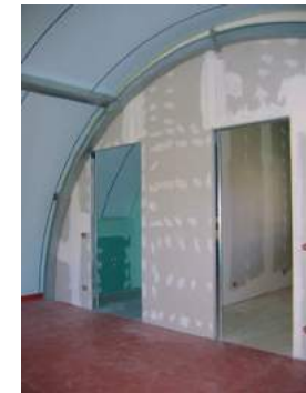
20. Inside plasterboard walls
