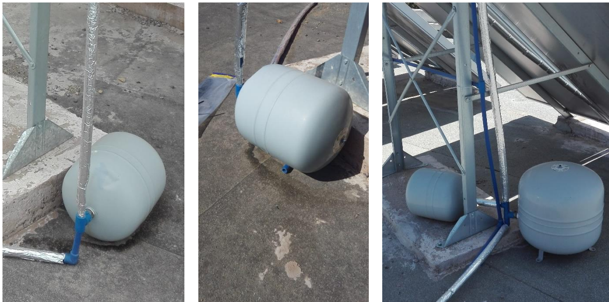
Figure 4.2: Expansion vessels placement.
