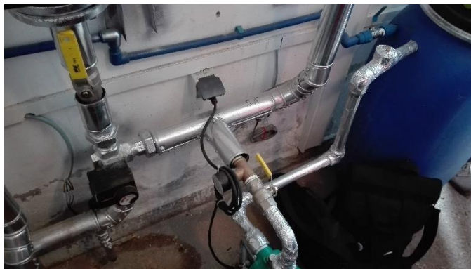
Figure 3.3: Internat Faidouzi, position of sensor S6 for bypass valve control.
