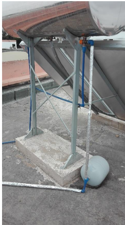
Figure 4.1: Domestic water pipes installation.
