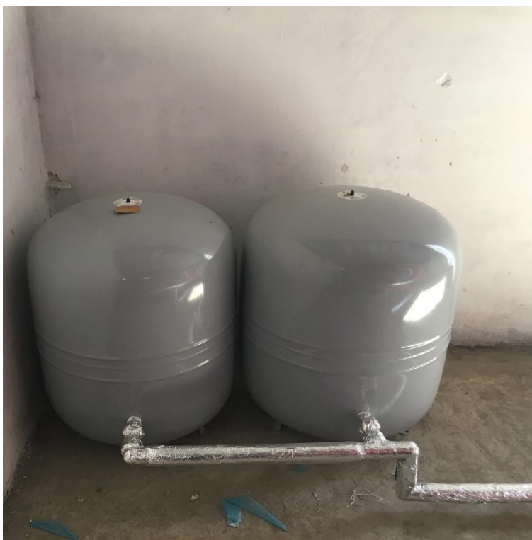
Figure 2.2: Cuisine Centrale expansion vessels, installed on domestic hot water side.
