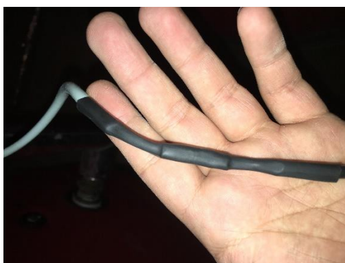
Figure 3.11: Protection of electrical connections.
