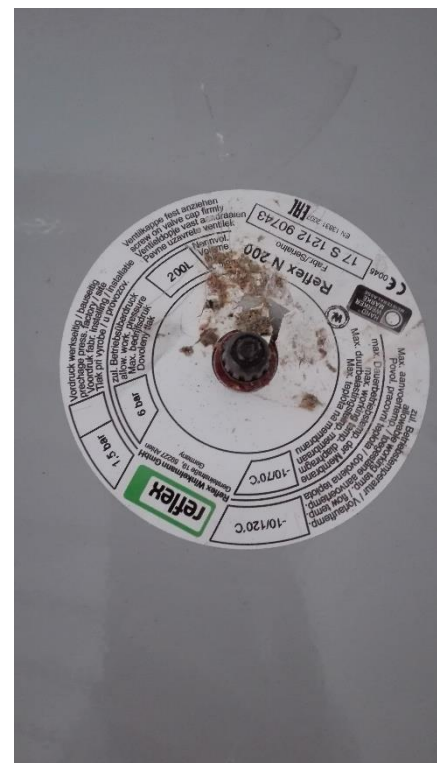
Figure 2.2: Cuisine Centrale expansion vessels, installed on domestic hot water side.
