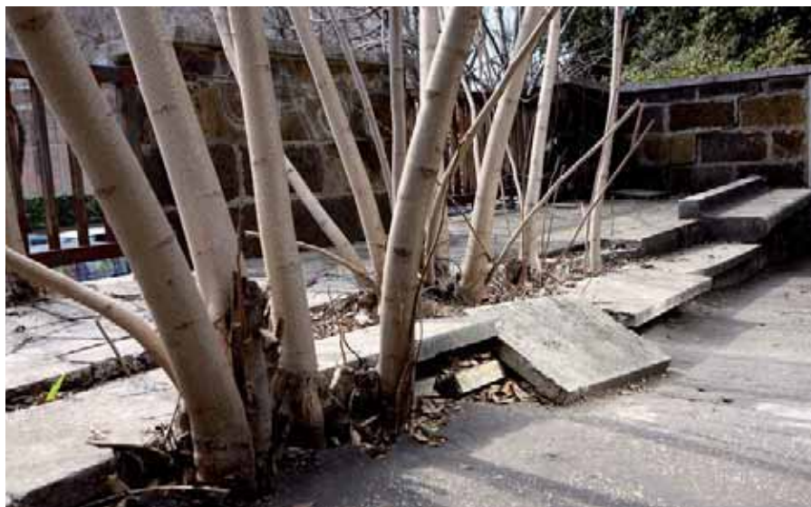
Ailanthus altissima , whose roots inflict serious damage on man-made constructions. Photo J. Grapow
