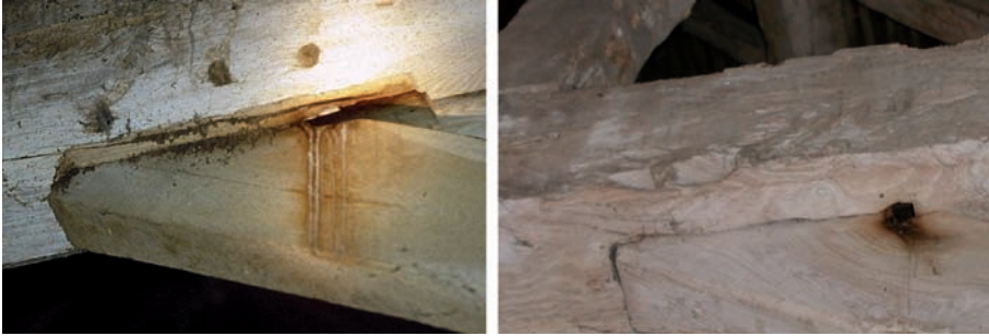
Figure 2.7 – Hollow mortice joints used by roosting bats in barns (after Briggs, 2004).
