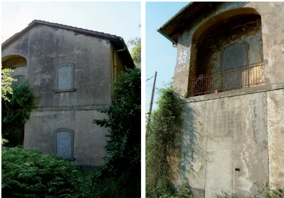
Figure 5.1 – Abandoned railway buildings – note walled up doors and windows.
